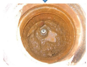
Inside the monument well there is a 3/8 inch iron pipe with a brass tag.
