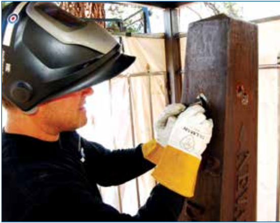
Cividino preparing to fill a large bullet hole on the monument's south face, June 17, 2014. Author's photo.
