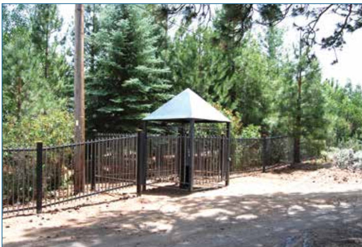
Fence and enclosure in place, June 14, 2014. Author's photo.
