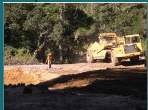
Construction staking for roadway and wellness facility improvements, Cazadero, Sonoma County.
