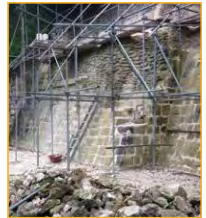
A temple under reconstruction.
