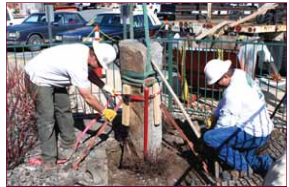
NVEnergy workers re-set the column at Boomtown.
