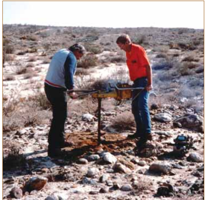
Then Party Chiefs Norman Peet (County of SD) and Ron Dodds (City of SD) auger to install a Bernsten rod type monument in the Eastern San Diego County desert
