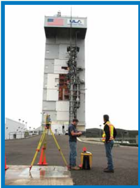
Space Launch Complex 3 on Vandenberg AFB. Pictured are James Walsh, LSIT and Justin Height, PLS. Submitted by: Justin Height, PLS.
