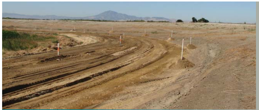
Fill markers are used to control thickness of lifts during construction.
