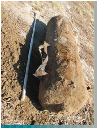
Abandoned fuel tank found and removed during levee rehabilitation.
