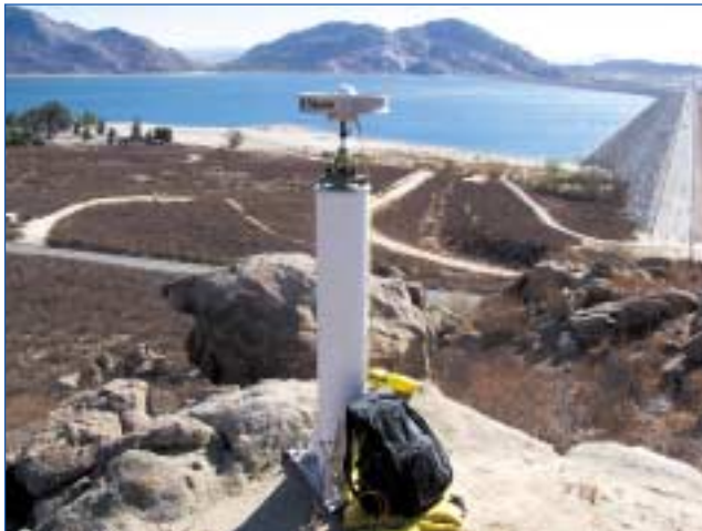
Pillar at Perris Reservoir. Control pillar overlooking Perris Dam in Southern California. Pillars of this type are installed in arrays around SWP dams for use in monitoring dam deformation.
