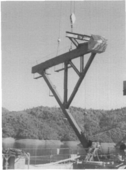
A temporary rigid frame and dam connector being craned into position.
