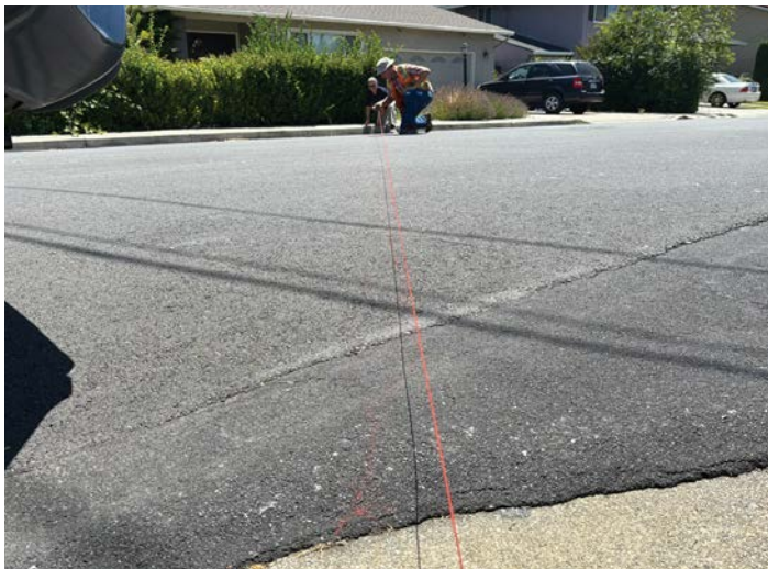
Snapping chalk to reset the point.
